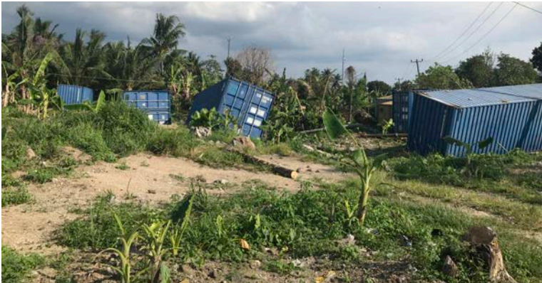
Fig. 21. West Java coast. Shipping containers used as condominiums (inside lined with brick) scattered 200 meters inland by the tsunami.
